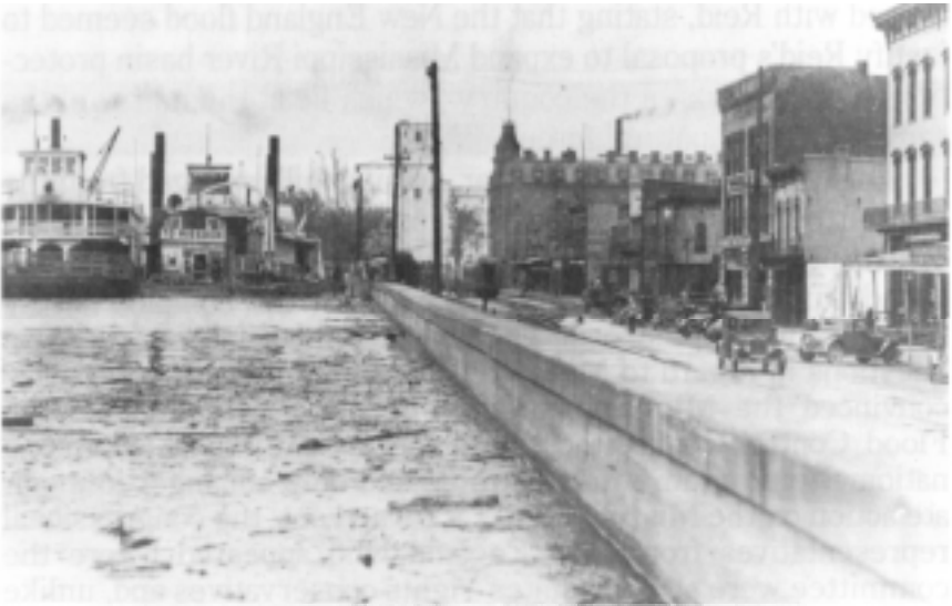
Floodwall at Cairo, Illinois, during the 1927 flood.
