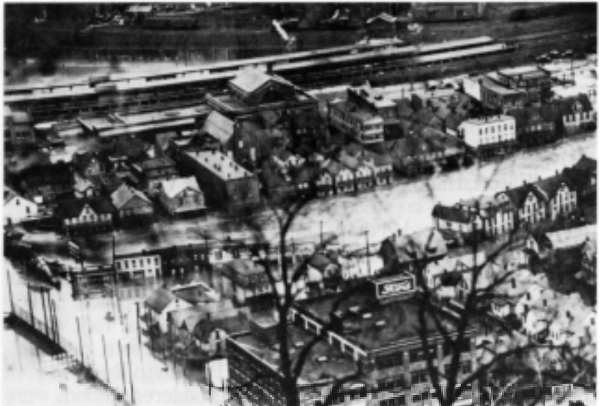
Johnstown, Pennsylvania, during the 1936 flood.
